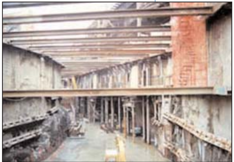
Excavation along side the in service Northern Boulevard Subway Structure.
