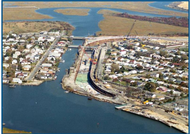
*During construction of the 2,900-foot long tunnel/depressed roadway section of the Atlantic City-Brigantine Connector, a shallow penetrating dewatering system ensured a dry excavation while minimizing offsite groundwater drawdown.*
