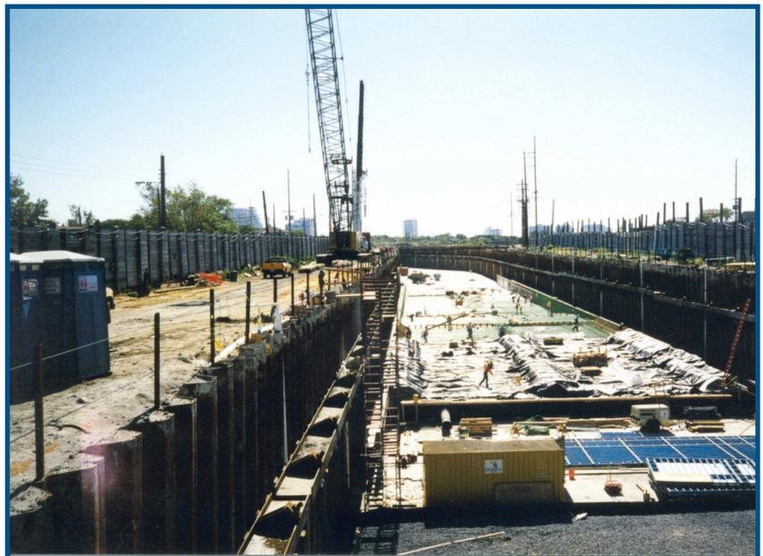
*The 100-well system was installed inside of the excavation support and operated continuously for the 16-month construction period.*
