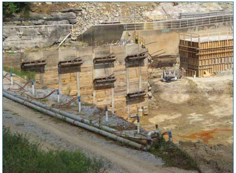
Top: Remediation of Bear Creek Dam involved excavation for the construction of a roller compacted structure at the toe of the existing dam.
