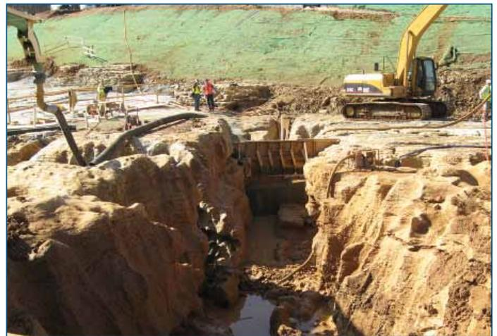
Top: Piezometer data showed that the total system pumped as much as 4,000 gpm at times.
