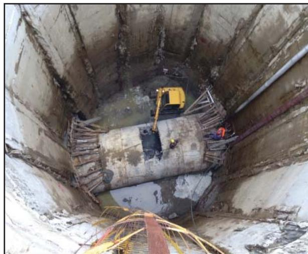
► Removal of the portion of the tunnel within the shaft prior to installation of the final concrete liner.
