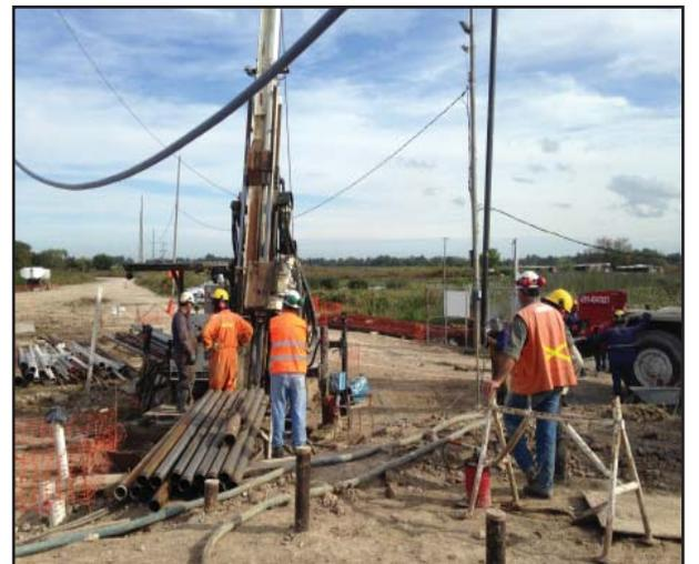
► Drilling underway for freeze pipe installation.
