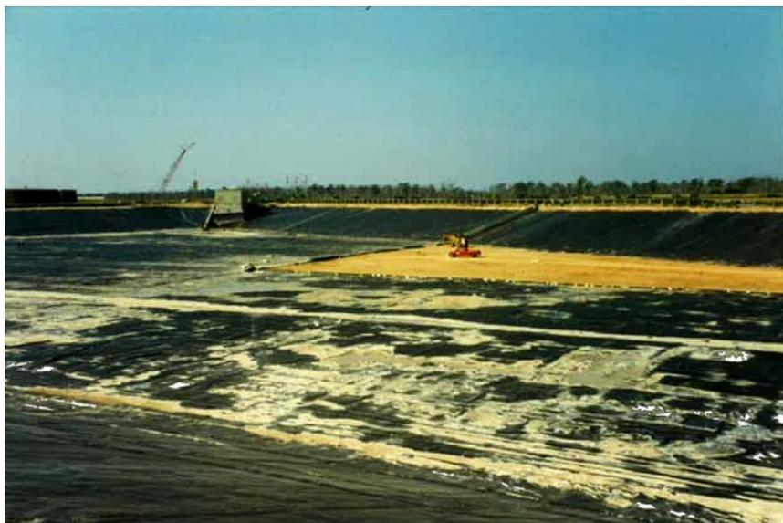
Figure 10: The pond is completely excavated and the HDPE liner is being installed.
