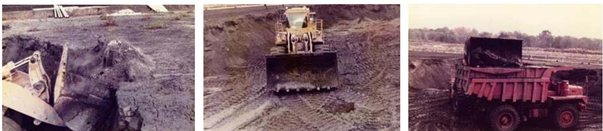
Figures 6a, 6b, 6c: Excavation of fly ash with rubber tire equipment.
