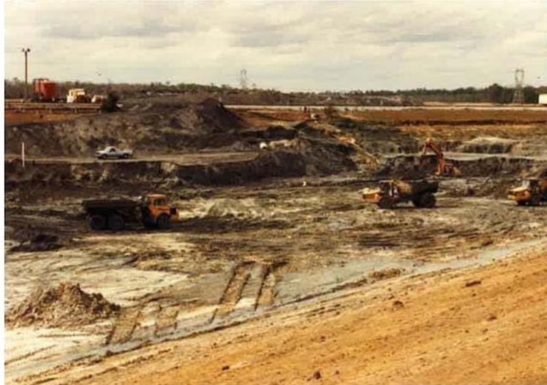
Figure 11: Excavation of the Plant Daniel pond. Because the ash is adequately pre-drained, it does not need to be removed in thin lifts.
