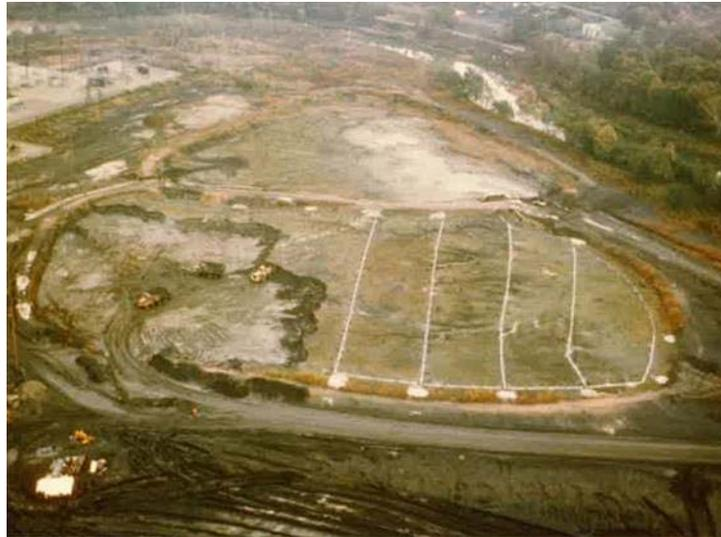
Figure 5: Partially removed system with excavation underway. The white wellpoint header is visible around the perimeter and across the pond.
