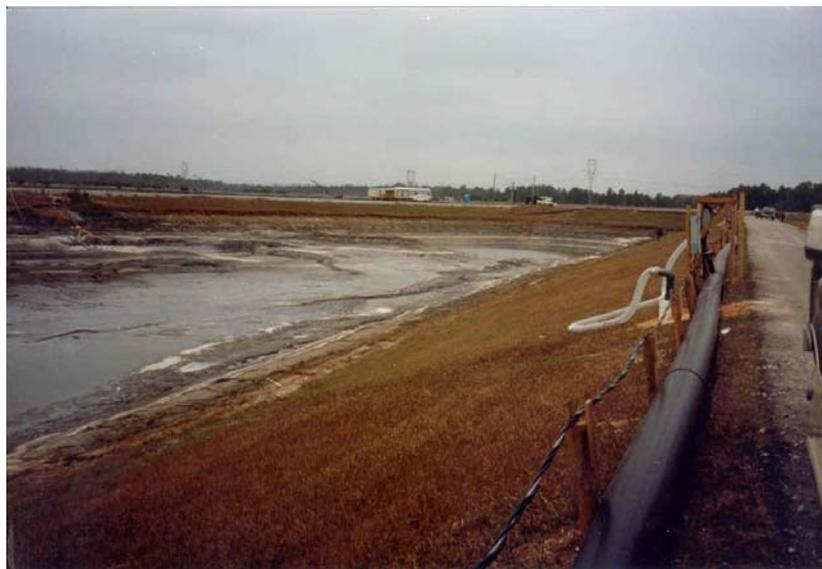
Figure 8: The pond was dewatered with a perimeter well system. The wells and discharge piping can be seen just inside of the perimeter road.
