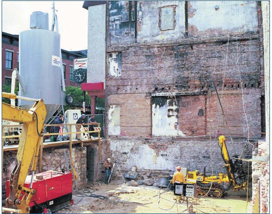
*Jet grouting was accomplished from the top of the footings to be underpinned.*
