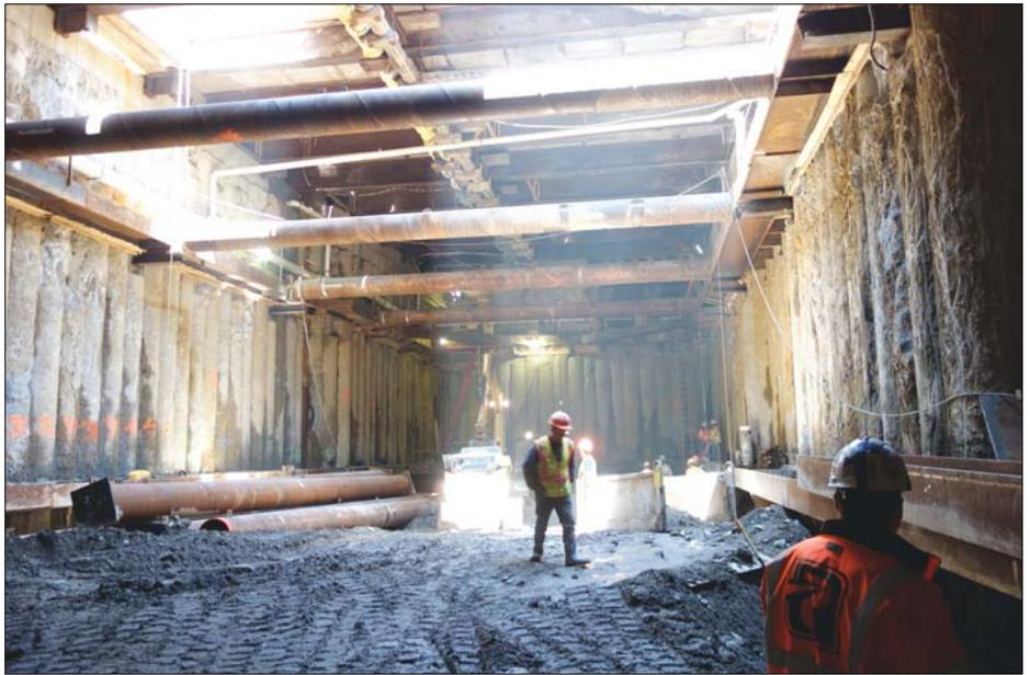
Figure 1. A permeation grout curtain was extended beneath the secant piles to rock. This enabled the vent shaft to be excavated to subgrade (pictured) in the dry.
