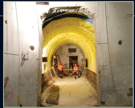
**Figure 11: Cross passage excavation**
