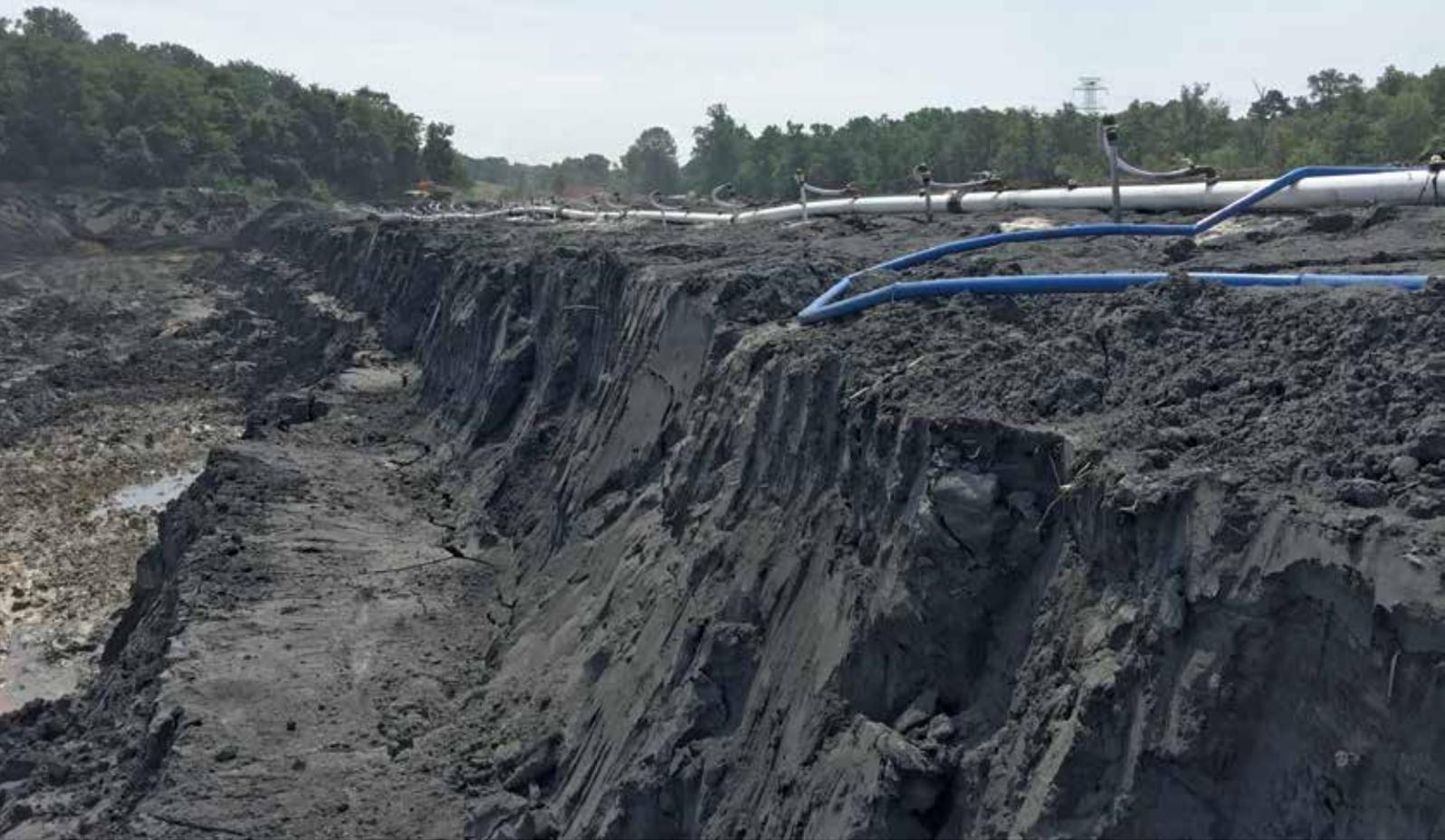
**Fig. 3: Wellpoint pre-drainage dewatering. Ash removal began approximately 5 weeks after groundwater pumping was initiated and completed 5 weeks later.**
