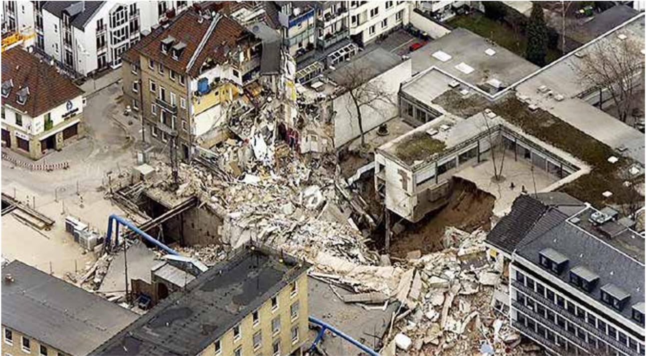
**Figure 3.** The scale of the 2009 collapse of a six-story archive building and two neighboring apartment buildings in Cologne, Germany, is evidence of the powerfully destructive effects of soil erosion with groundwater flow. (Photo courtesy of TunnelTalk.)
