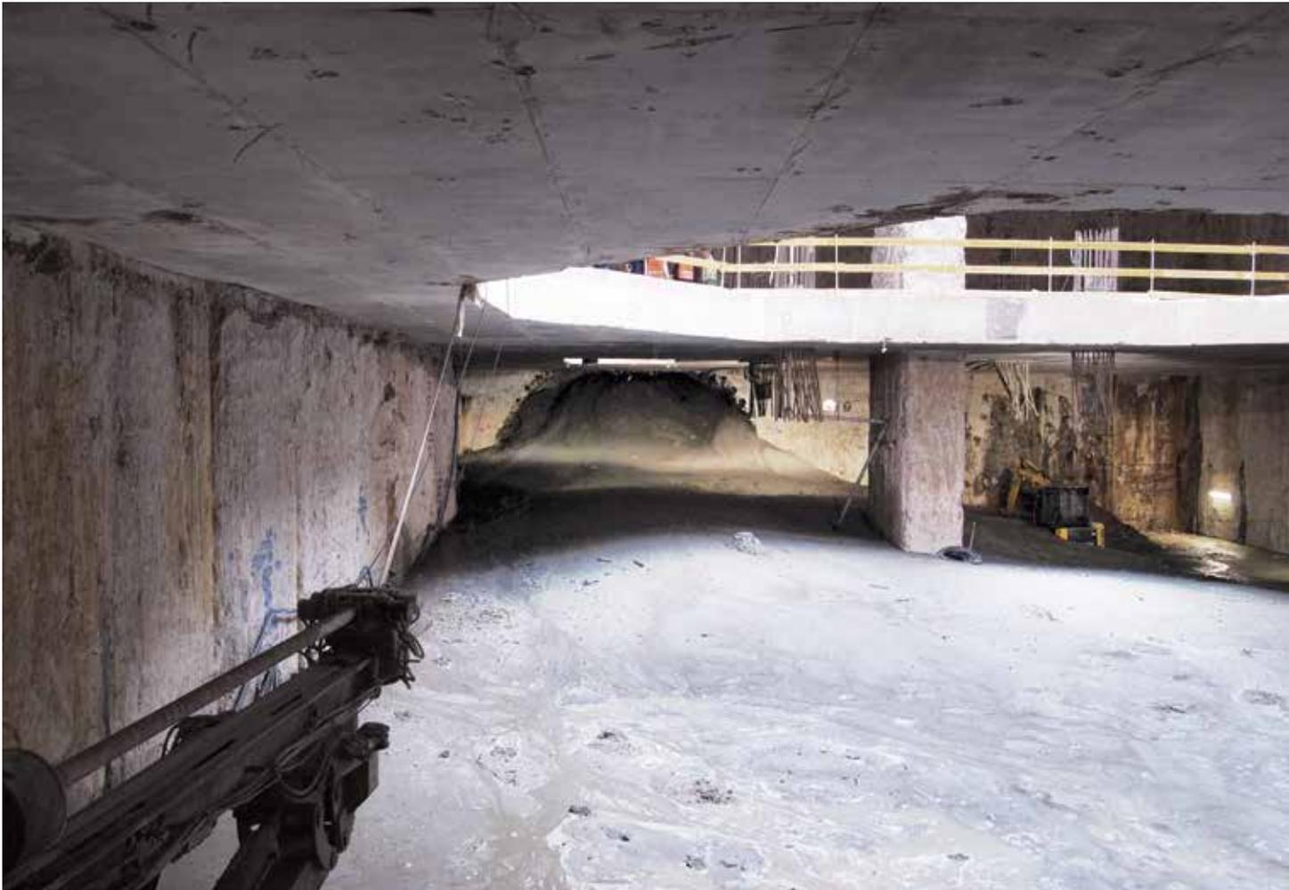
**Figure 5.** Post-failure conditions following collapse of jet-grouted soil canopy during construction of a tunnel at the Powisle Metro Station in Warsaw, Poland. An imperfection in the jet-grouted canopy caused significant ground loss. Note the buried equipment in the right side of the photo. (Photo courtesy of Metro Polska.)
