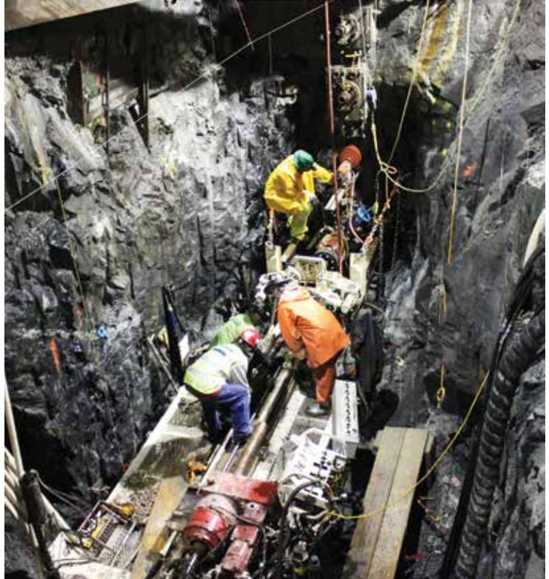
water table. However, given Moretrench's experience of drilling and working with difficult Bull's Liver-like soils below the water table, particularly on the adjacent East Side Access section, there was every indication that this approach would be viable, should it be required. A secondary arch of heat pipes was also incorporated to control the outward growth of the freeze.
